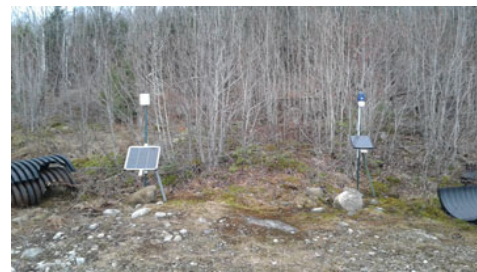
Fire sensors. Photo: Government of Canada
