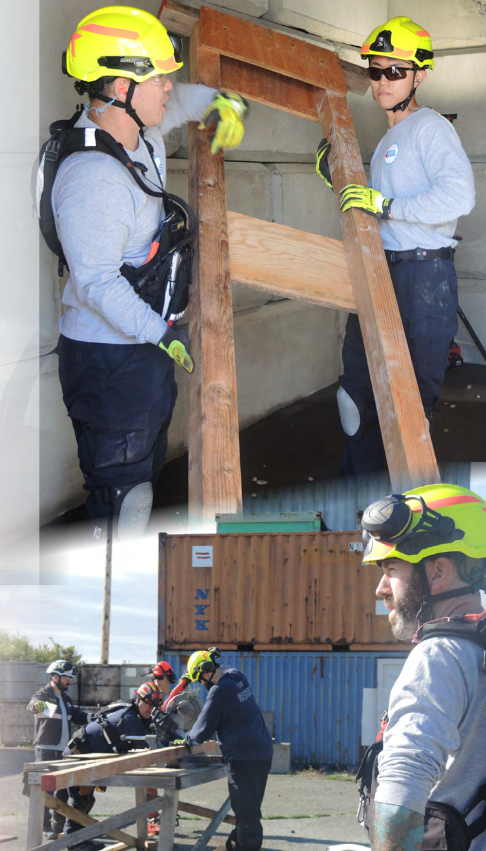
Members of the Vancouver Island MUSAR team erect wood shoring to stabilize a partially-collapsed structure during a training exercise on July 31. Photos supplied.
